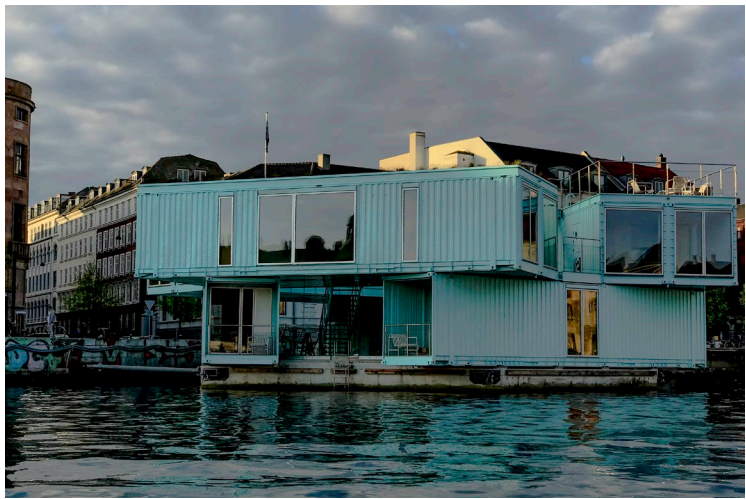
Floating container student homes “Urban Rigger” by the Bjarke Ingels Group, Copenhagen. Source: Jimmy Baikovicus, Flickr.
