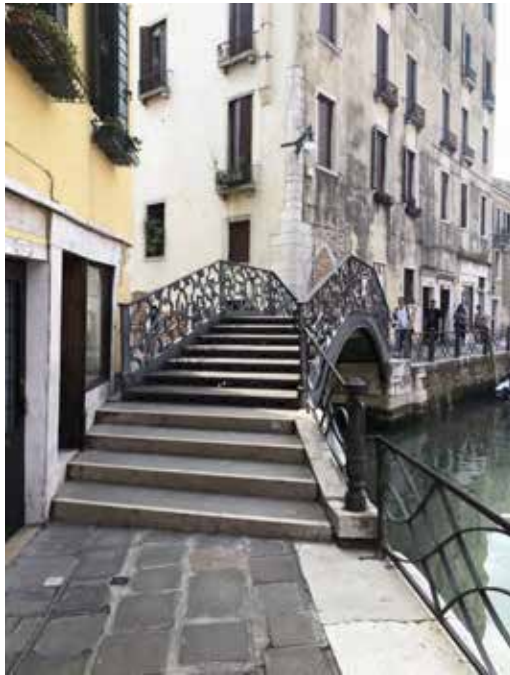
Figure 5. (Left) Example of a bridge with an iron rail. The top of the rail is used as a support by the elderly both up and down the steps as it allows for good grip. (Right) Example of a bridge with a brick wall and added handrails on both sides.
