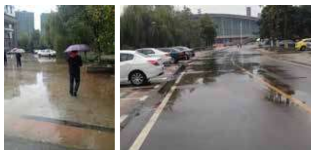
Figure 8 Water accumulation in impervious pavement
